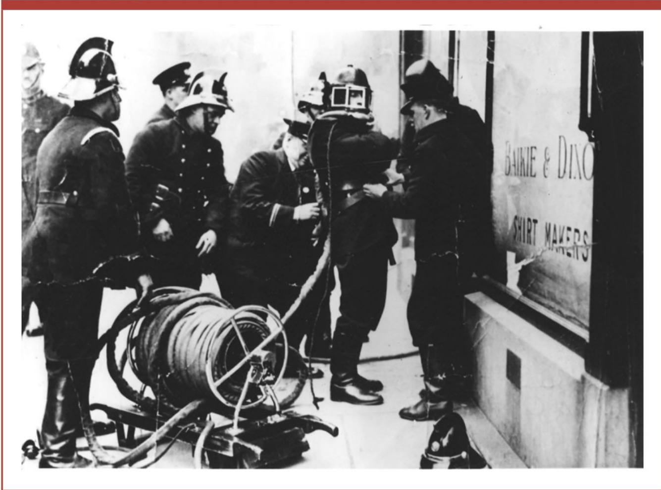
Figure 3.1 A tethered helmeted fire fighter prepares to enter a structure. (Source: Photograph from the Scottish Fire and Rescue Service Heritage Trust.)
