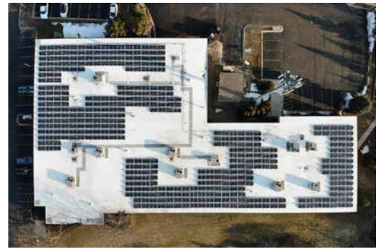
Installing solar panels at HQ has already saved 845,000 lbs. of CO2 emissions and will save thousands of dollars annually, after five years.
